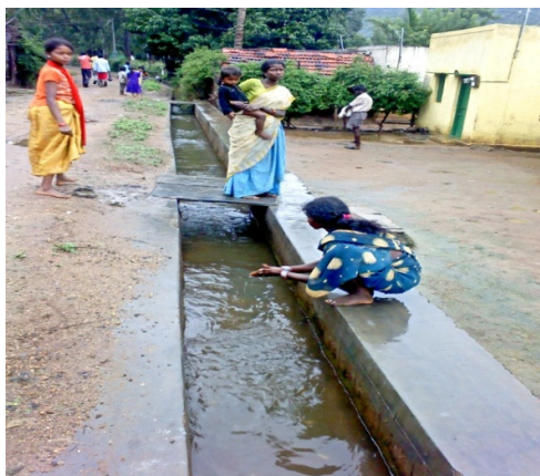
A small canal at Kowlihalla dam
