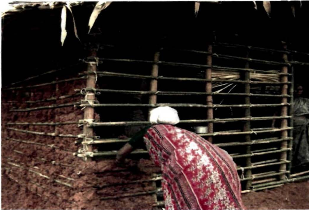
Picture 1. Muthuvans building a house with mud and bamboo sticks
