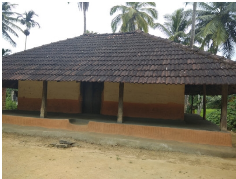
Figure 5: The daivappura in the Kuranjuvayal Kuruma settlement in Pulpally Panchayath, Wayanad
