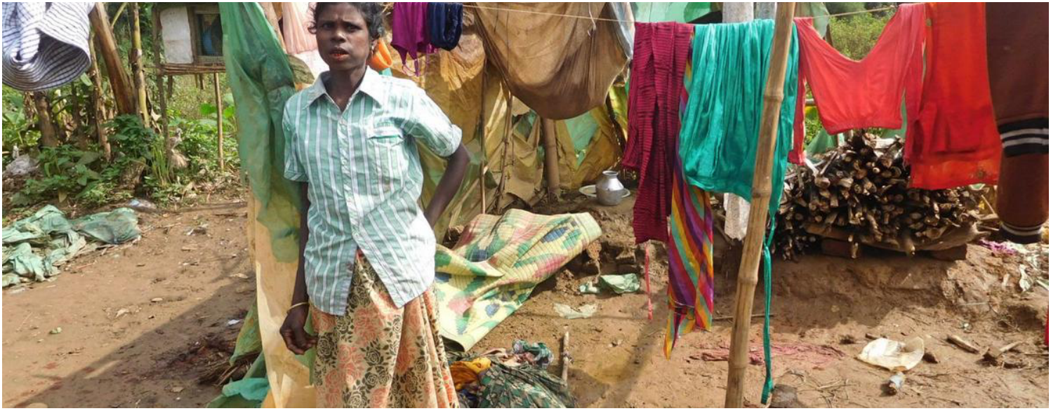
Bindu (in photo) and her husband Gopalan live in this damaged shelter in Wayanad's Venniyode Vaishyan Adivasi Colony after the floods. | TA Ameerudheen
