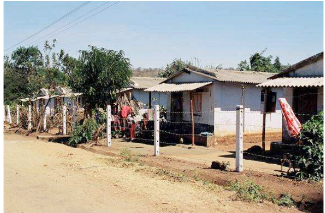
Figure 19 Adivasi houses constructed by the government, Eruru village The corrugated iron roofing of these houses is completely unsuitable for (semi)tropical climates (9. focus group interview 2007). Photo: C.C. Aufschnaiter
