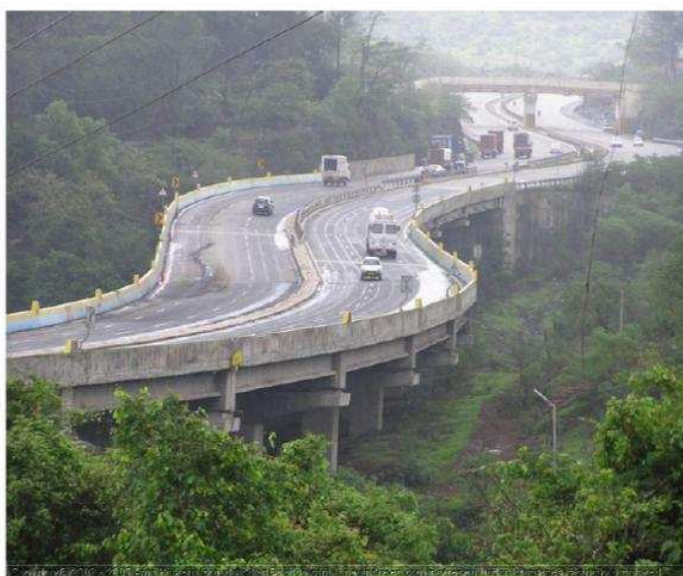
Figure 12 The Mumbai-Pune Expressway Courtesy
